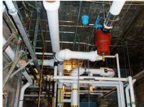
Air separator and automatic air vent.
